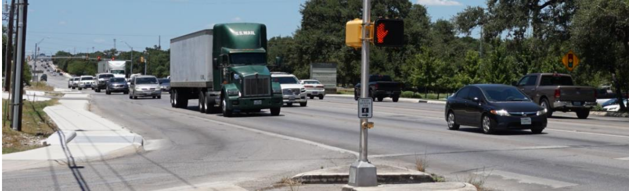
Roy Richard Drive, with recent sidewalk improvements
