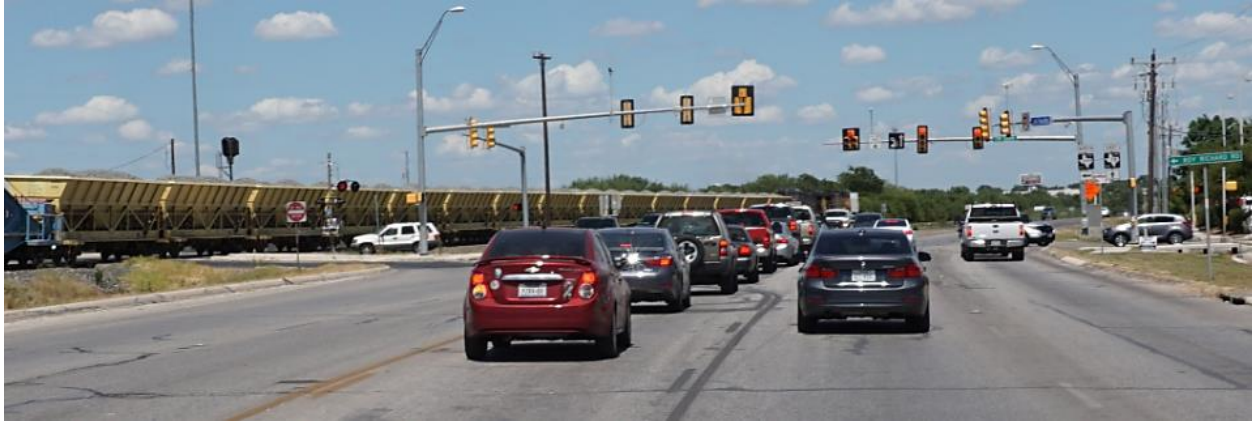
Traffic stopped for train – intersection of FM 3009 and FM 78. Illustrates the confluence of transportation modes needed to maintain mobility and connectivity in central Schertz despite increasing travel demand and rail disruption.
